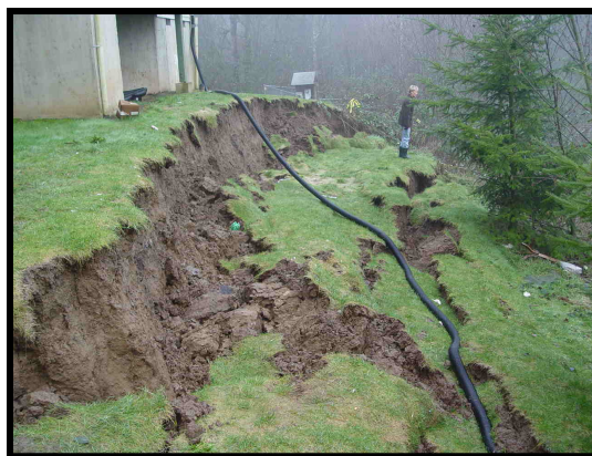
Landslide in Portland, 2006. An apartment house, built on a site which geologists recommended against, began moving when the old landslide reactivated. Oregon City, Oregon. Photo by S. Burns.
