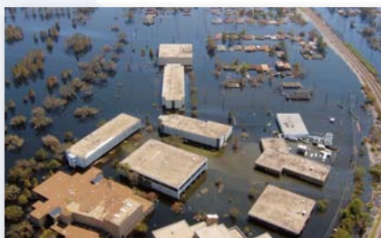
Flooding in New Orleans, 2005.
