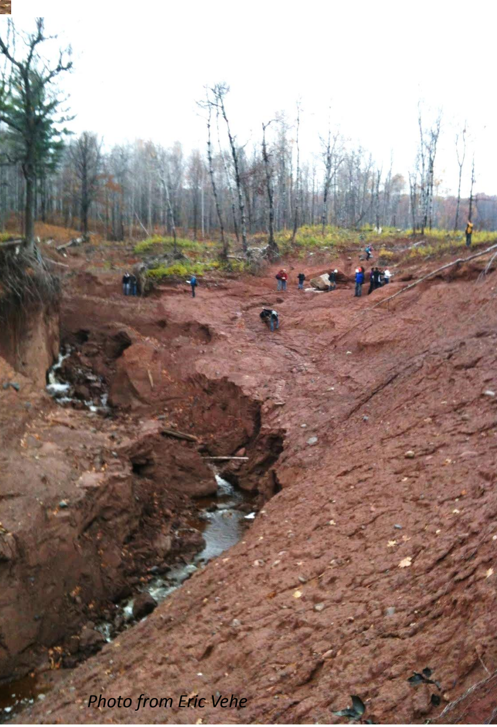
Levee breach as viewed from above (top) and from the ground (left). The failure occurred rapidly, sending a wave of water and sediment downslope.
