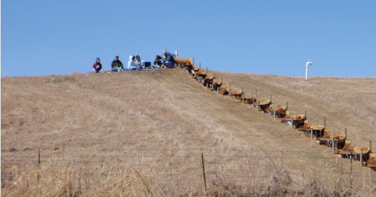
Students working at the top of the cascade aeration system where pumped water emerges from within the closed landfill.
